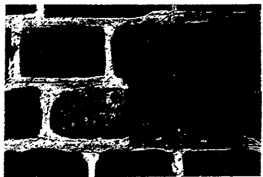
Palmer House, built between 1756 and 1760. In later years it was put to various uses. Right. A view of the "putlog holes" of the Palmer House. (The holes left by scaffolding timbers were not filled with bricks when builders left the job and are now vacant.)
